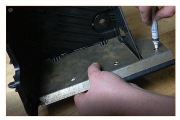
Attach the MM2356-02 bracket to the MM2356-01 degas tank using the 2x short 5mm allen bolts. Leave these bolts loose. (2x short 5mm allen bolts).
