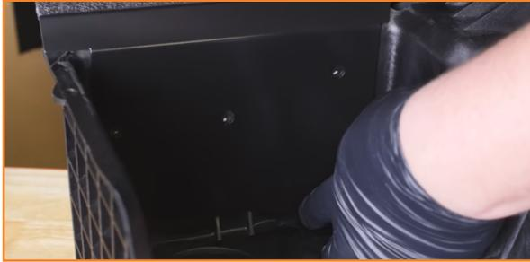
15. Using the three markings, drill holes through the battery box. (3/8" drill bit and drill)
